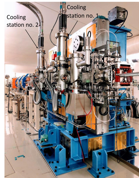
FIG. 1. TPS-CUT18 installed in the TPS storage ring.
